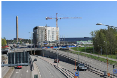
Figure 6. Photo of the Skanska building partly ready.
